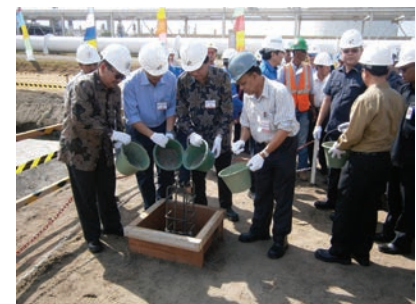
(Groundbreaking pembangunan Arun LNG Receiving Hub & Terminal Regasifikasi 9 November 2013) (Groundbreaking of Arun LNG Receiving Hub & Terminal Regasification on November 9, 2013)
